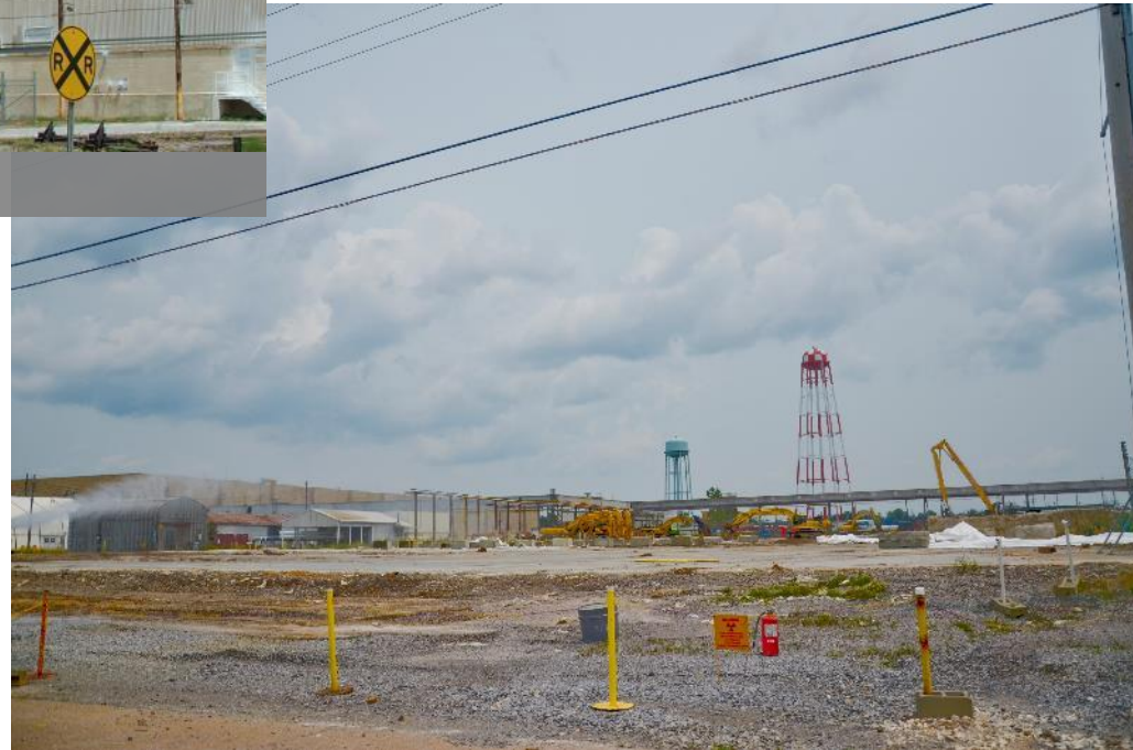
C-410 Feed Plant Demolished
